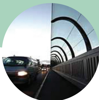
Grafton Bridge barriers, Auckland Photo: NZ Herald
